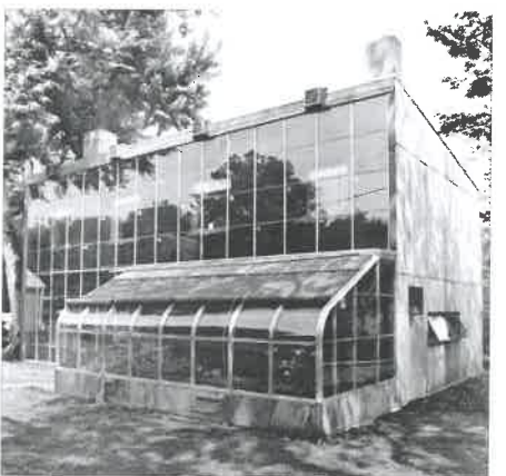
Douglas Kelbaugh, Haus Kelbaugh, Princeton / New Jersey, USA 1975, Foto: Robert Perron, aus: Louis Gropp: Solar Houses, New York 1978
